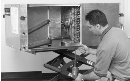
Figure 51. Install top/bottom filter rack
