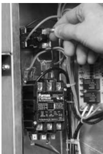
Figure 63. Connecting speed-tap wire
